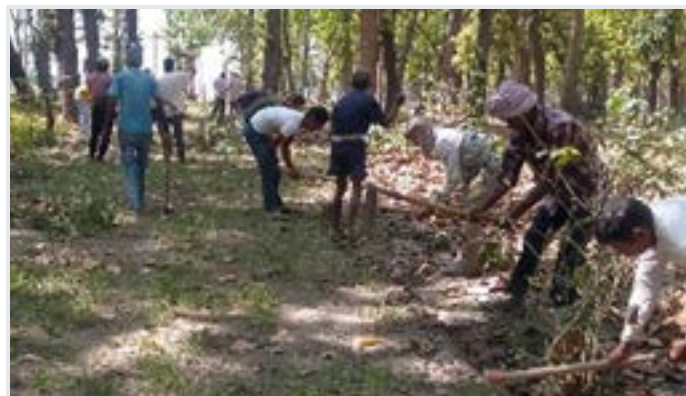
Constructing the fire lines.
