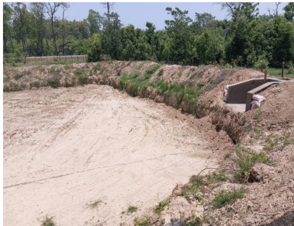
Figure 9 Constructed Outlet in Recharge Pond at Khaurahawa Shiv CFUG
