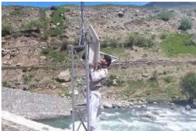
Checking of Data Acquisition Unit (DAU) in Pariyan district, Panjshir.
