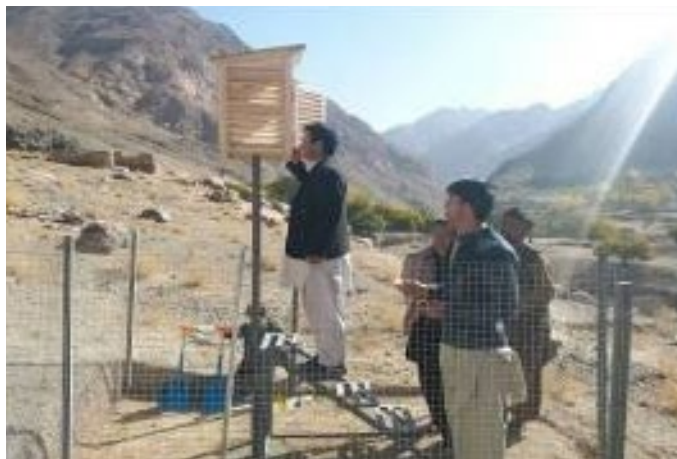
WMP installation in Baghlan province.
