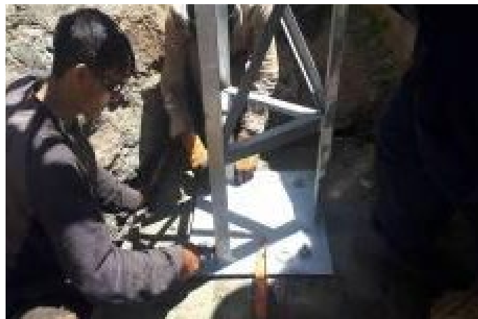
Installation of CBFWEWS pole in Pariyan district, Panjshir
