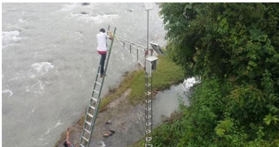
Installation of Sensor in the Kalakot area.
